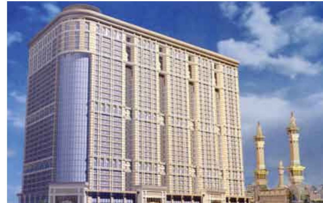
Bakkah Tower, Makkah - One of Munshaat Real Estate Projects Company K.C.S.C.'s Projects
